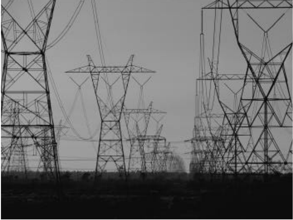
EPRI's communication and information sharing tools enable industry participants to link the trading, security, control, and dynamic data infrastructures together into a seamless network supporting the grid.
